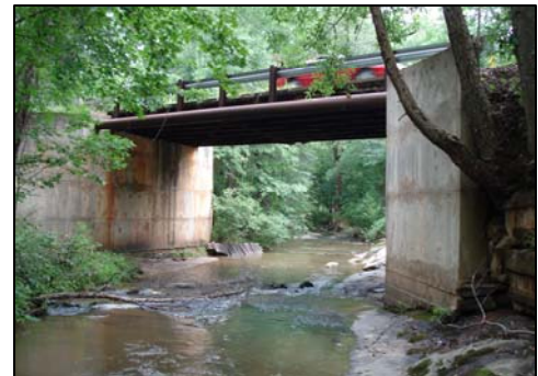
Zimmerman Road Bridge
