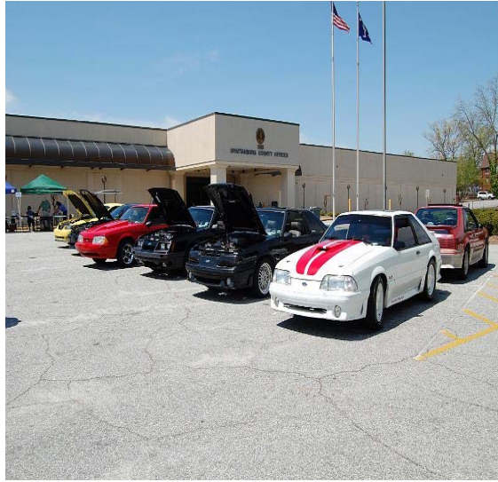
Spartanburg County Administration Building
