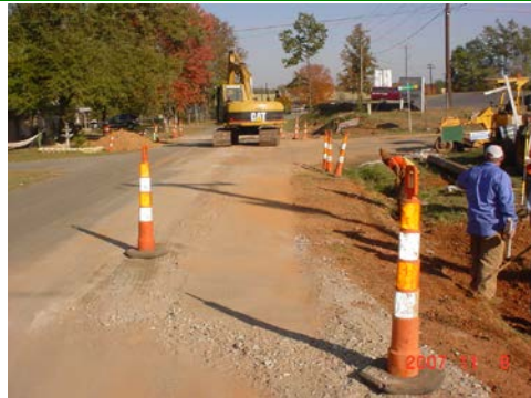
Water Project Construction
