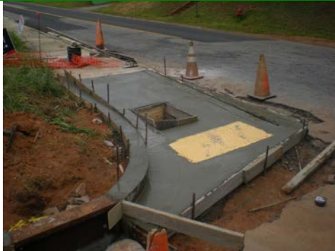
Repair Work on a catch basin
